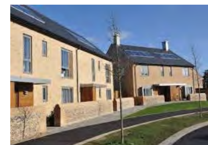
RENEWABLE ENERGY TECHNOLOGY CAREFULLY CONSIDERED IN STREETScape
