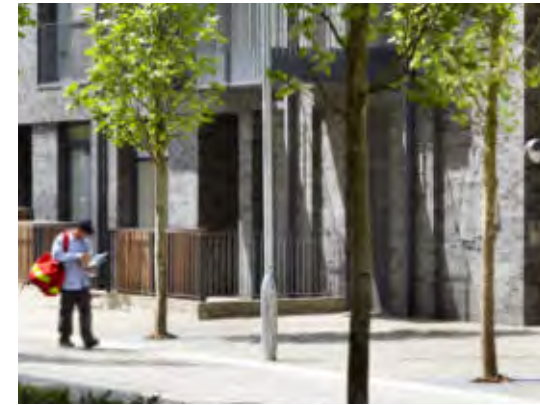
Apartments in an urban setting, with street entrances
