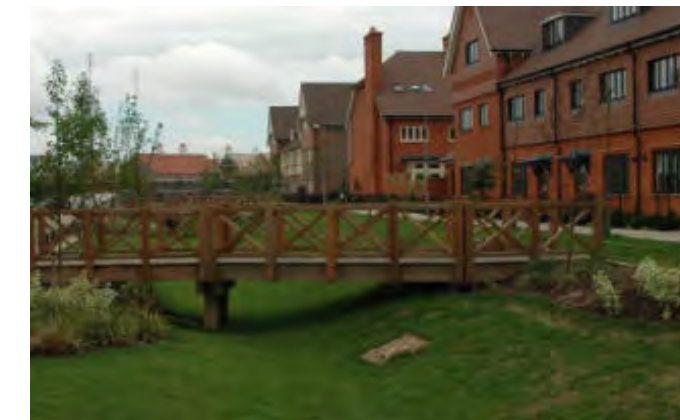
Simple dry swale running along street
